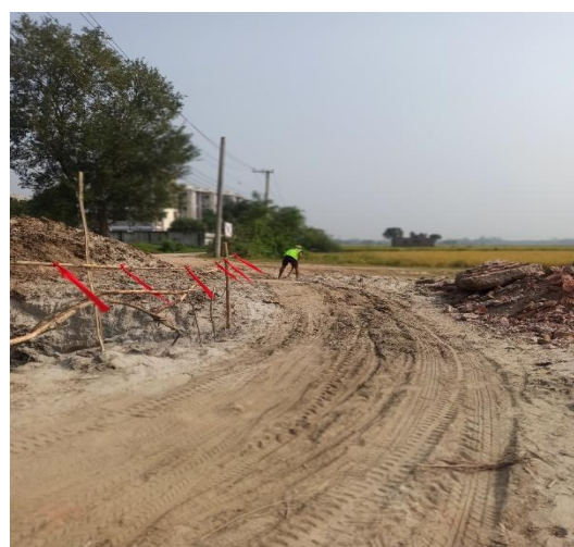
Temporary and alternative road at the Culvert area on November 18, 2024
