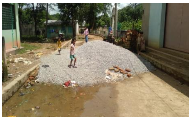
During first visit: no space for movement of people
