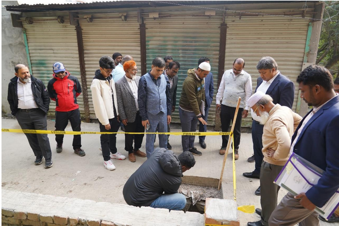
Figure 20: The ADB and AFD Review Mission is checking ongoing IUGIP works at Naria
