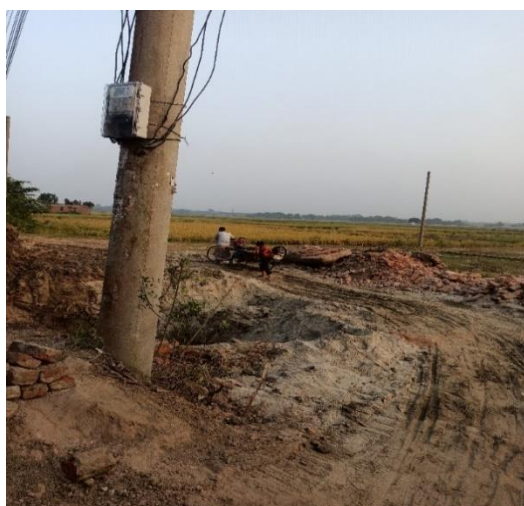
Temporary and alternative road at the Culvert area on November 17, 2024
